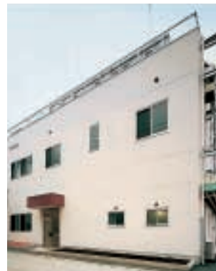
View of the research and development building (Sagami Operation Center)
