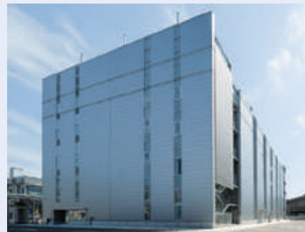
New C-1 Building of the Sagami Operation Center, where R&D is promoted in cutting-edge areas centering around the super clean room to handle hazardous substances
