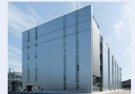
New C-1 Building of the Sagami Operation Center, where R&D is promoted in cutting-edge areas centering around the super clean room to handle hazardous substances
