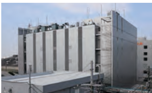
New R&D Building at the Sagami Operation Center
