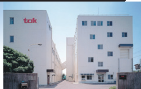
Shonan Operation Center
