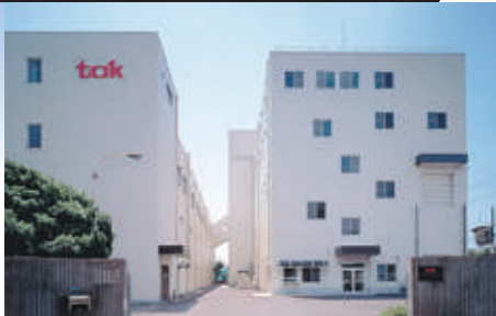
Shonan Operation Center
