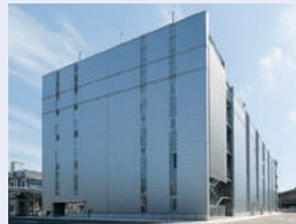
New C-1 Building of the Sagami Operation Center, where R&D is promoted in cutting-edge areas centering around the super clean room to handle hazardous substances
