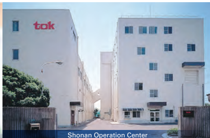
Shonan Operation Center
