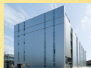
TOK Technology and Innovation Center (TTIC)
