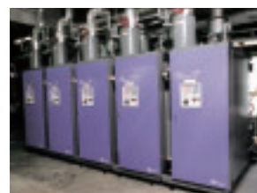
Natural gas boilers (Sagami Operation Center)
