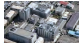
Sagami Operation Center/New R&D Building
