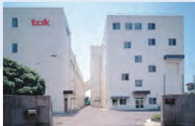
Shonan Operation Center
