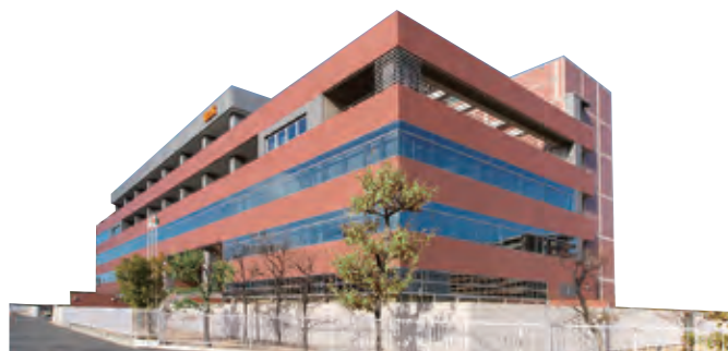
Tokyo Ohka Kogyo Co., Ltd., Headquarters
