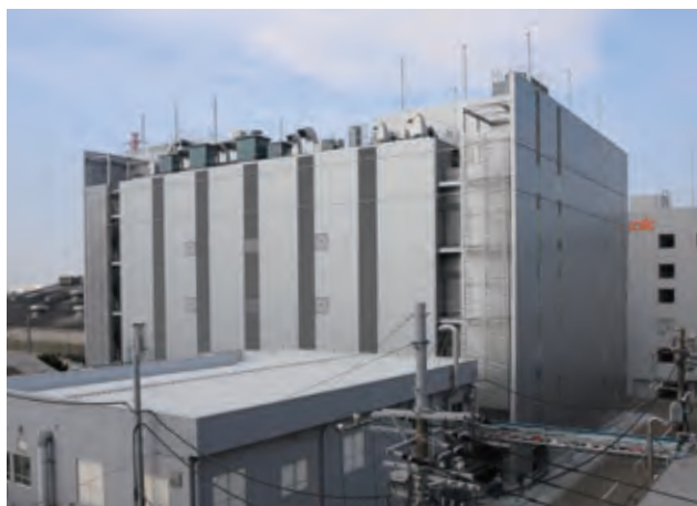
New C-1 Building (under construction) at the Sagami Operation Center will have a super clean room
