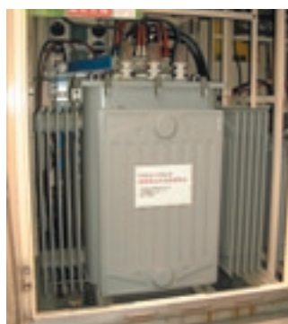
Electrical substation facility at the Sagami Operation Center, where PCB contamination was found
